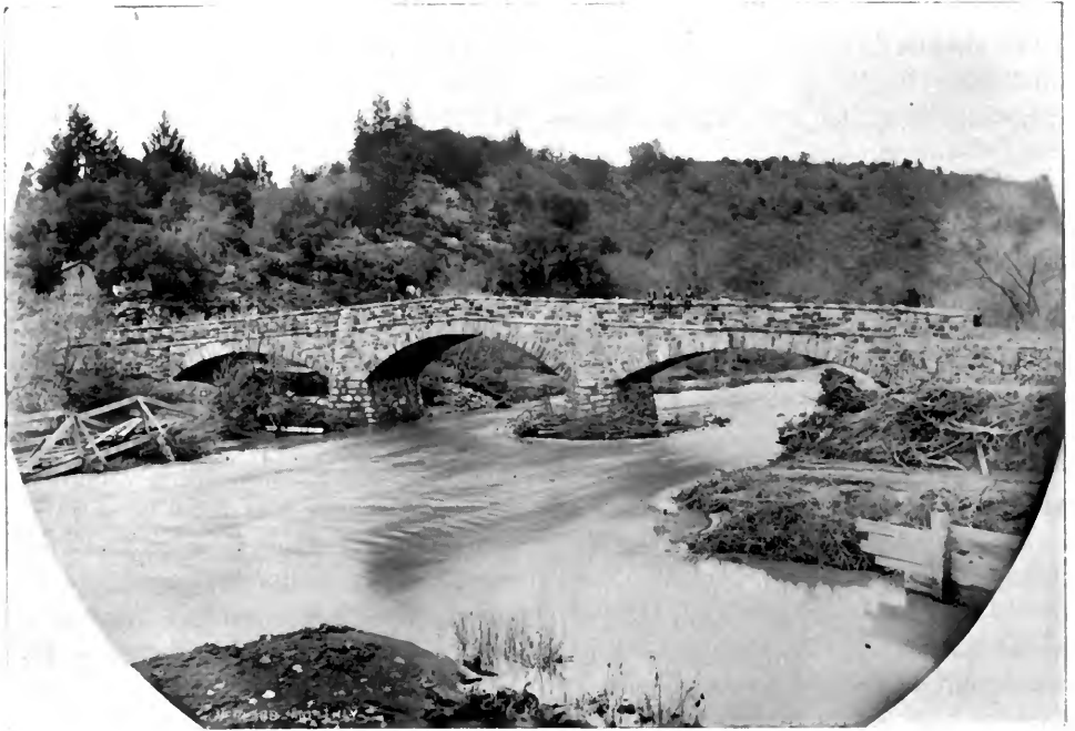
STONE BRIDGE WITH THREE FIFTY-FOOT SPANS, ACROSS NAPA RIVER AT ST. HELENA.
